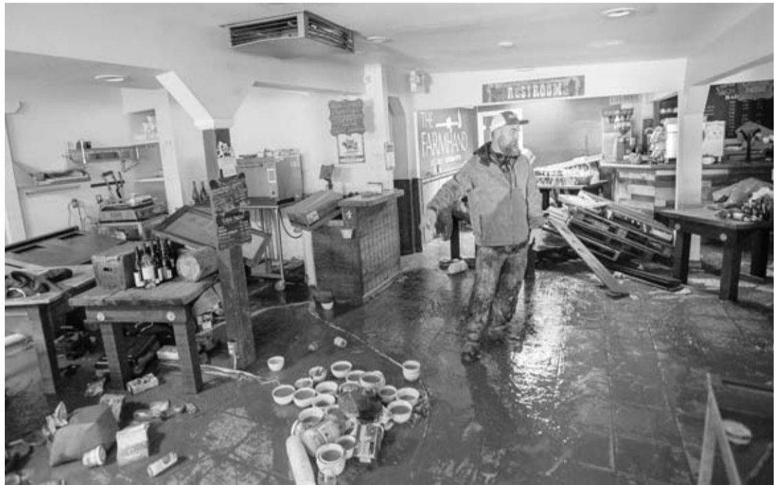
Farmhand Deli co-owner Jason Flint surveys the damage inside his restaurant along River Road as flood waters from the Russian River continue to recede in Guerneville, Calif., on Friday, March 1, 2019.
